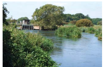
Fish counter and flow gauging weir across the River Frome at FBA East Stoke.
