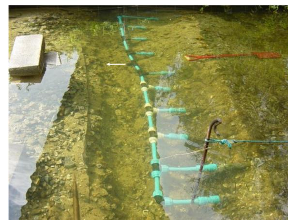
Fig 5. Hyporheic water collection manifold (30cm depth below gravel) prior to connection to a single through-riverbank pipe (arrow) and burial
