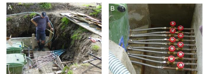
Fig 6. a) Connecting and concreting in downwelling pipes; b) downwelling pipes, flow control valves and a collection reservoir
