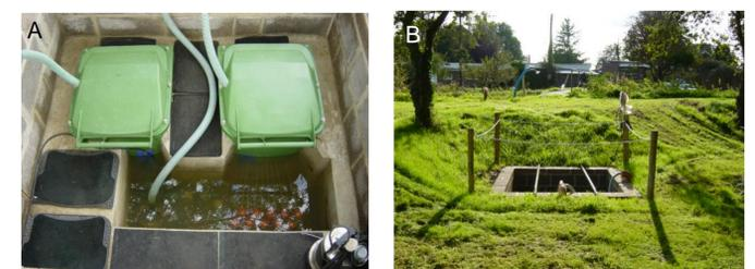
Fig. 7a) Completed collection reservoirs with main pumps installed; b) reinforced concrete chamber housing collection reservoirs and pumps
