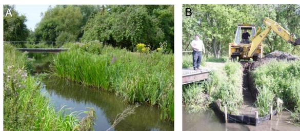
Fig 3. a) Study site on the Mill Stream, Dorset, England; b) Excavation of a sub-streambed depth trench through the stream bank
